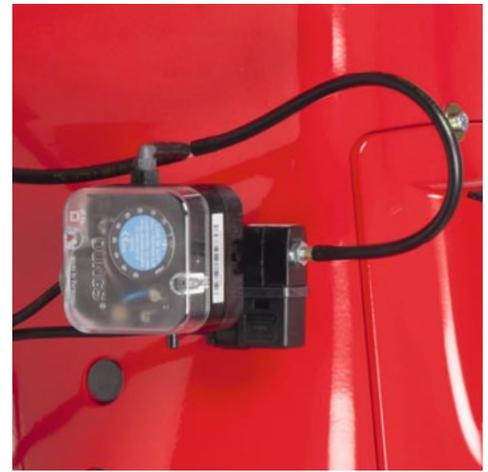
An additional solenoid valve enables the W-FM to also test the air pressure switch on burners with a post-purge or continuously running fan facility, ensuring maximal safety
