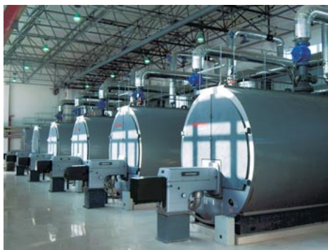
Xi'an, central China: The seven WKG gas burners in this heating centre provide more than 50 000 residents in the Zi Wei garden district with 115 MW of heat
